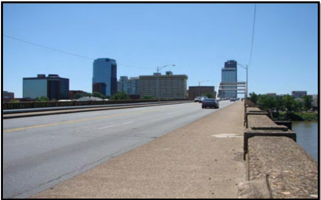
Figure 18. View to the south on the Broadway Bridge
