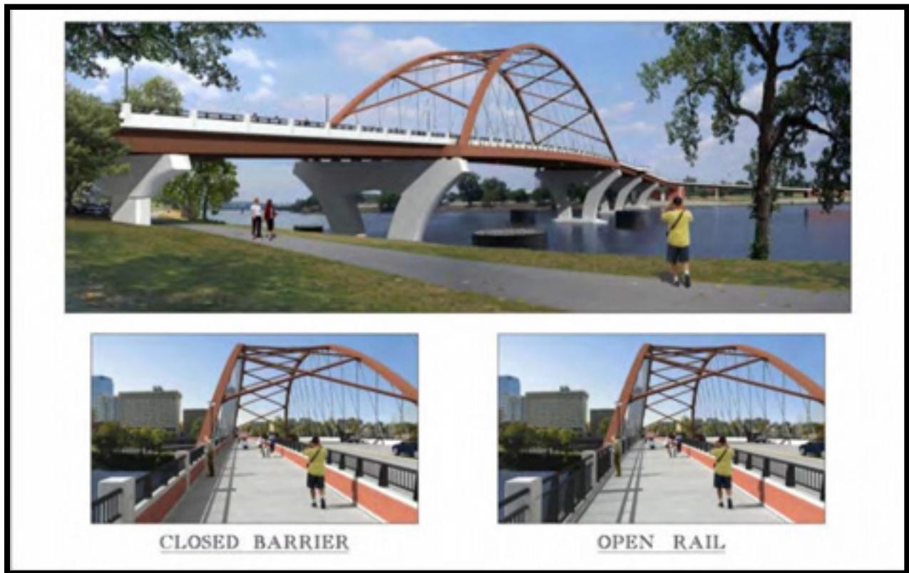
Figure 4. Single Tied Arch Bridge with Five Lanes and a 16-foot Shared Pedestrian/Bicycle Facility
