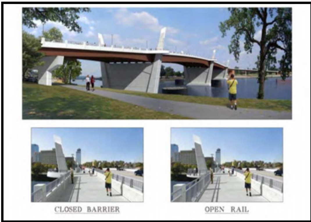
Figure 10. Plate Girder Design Bridge (Contemporary Design)
